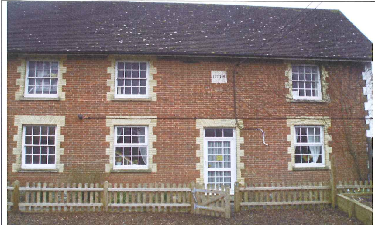
View of the North West Elevation, indicating area for the new access ramp and automatic entrance door to main reception area.
