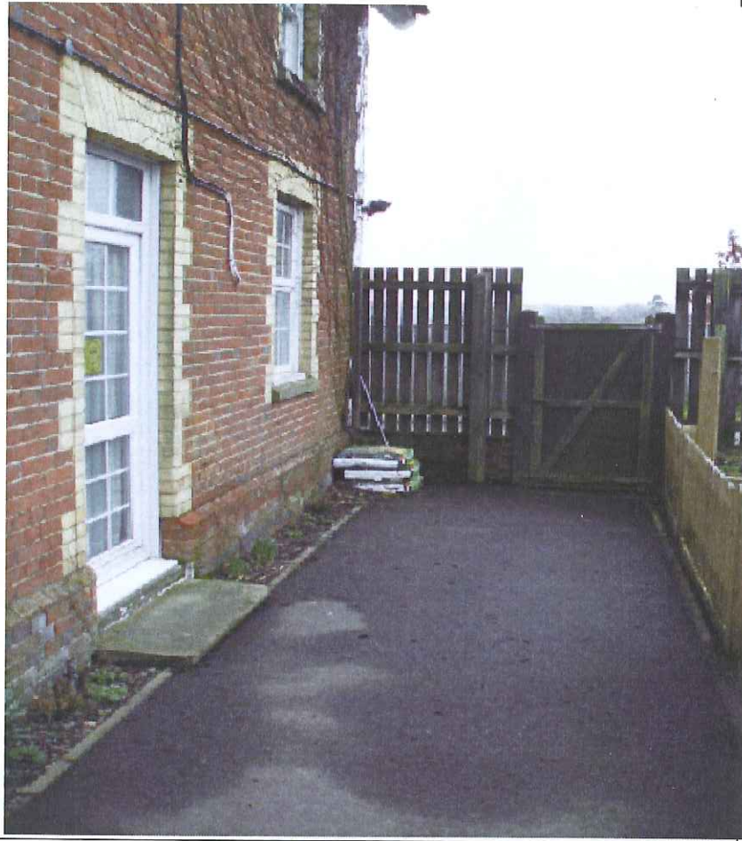
View looking down the North West Elevation, indicating area for the new access ramp and new security entrance gate
